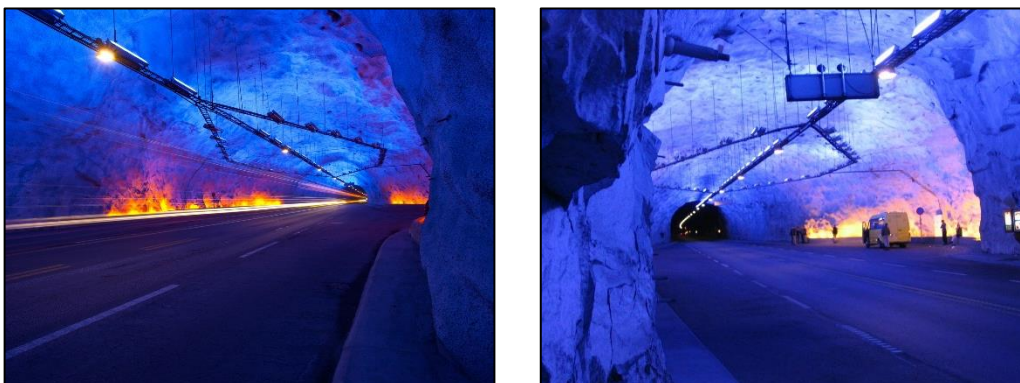
Figure 6-1 – Lærdal Tunnel lighting and cavern
